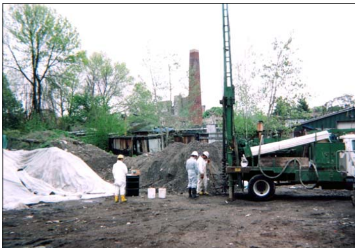
Soil boring and monitoring well installation at a Brownfield Site; PCB and Metals impacted scrap metal yard.
