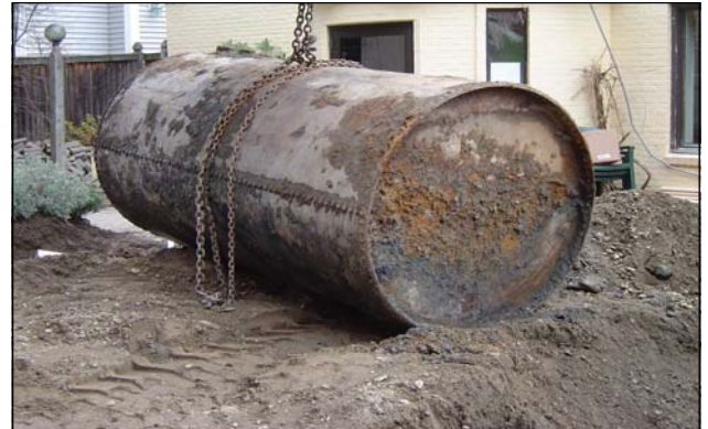
Leaking Underground Storage Tank removal.
