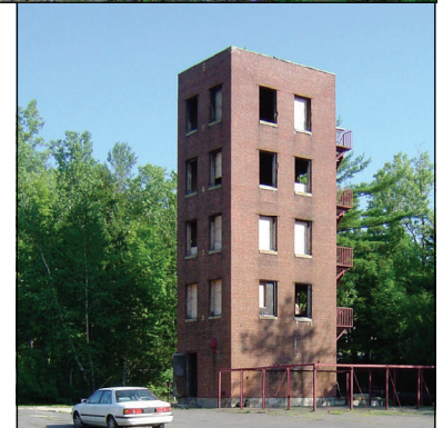
Five-story brick and concrete fire training tower with a basement built in 1951/52.
