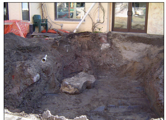
The UST grave after soil excavation and confirmatory sampling.
