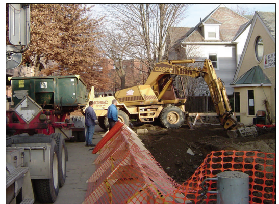
Excavation of oil-impacted soil into roll-off containers.
