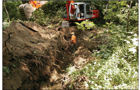
Test pits for soil characterization.
