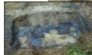
Removal of the drywell, an dry injection well, and associated sludge.
