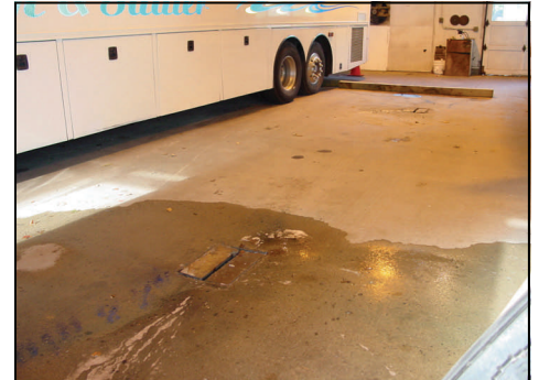
Garage floor drains and effluent pipe clogged with sludge.
