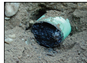
Garage floor drains and effluent pipe clogged with sludge.
