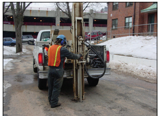
Limited Subsurface Investigation was conducted using a geoprobe drill rig and continuous soil sampling.
