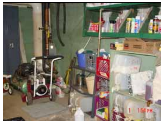
NEE inspected areas where oil and hazardous materials were stored, utility rooms, and all common areas of the facility.
