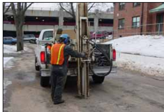
Limited Subsurface Investigation was conducted using a geoprobe drill rig and continuous soil sampling.
