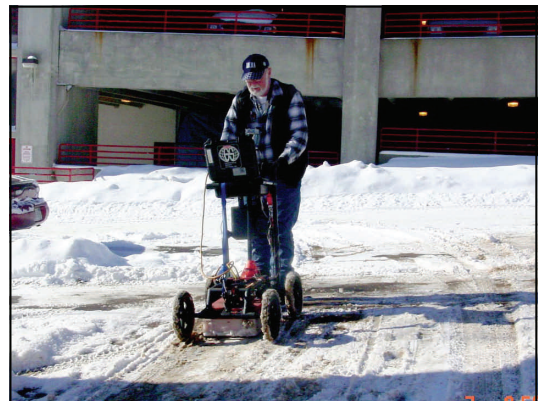
Ground Penetrating Radar (GPR) was used to locate historic underground storage tanks and current utilities prior to drilling.
