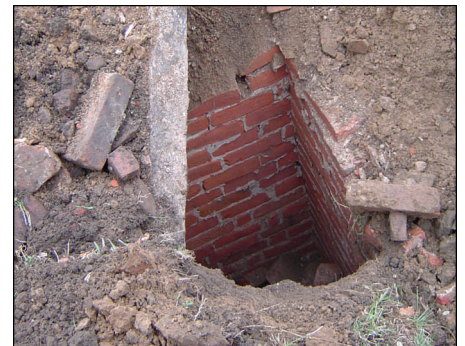
Foundations remain below grade at the Site.
