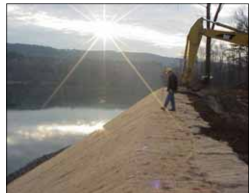
Re-graded bank with biodegradable erosion control blanket installed.
