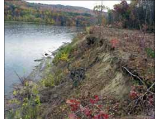
Eroded bank prior to site excavation.
