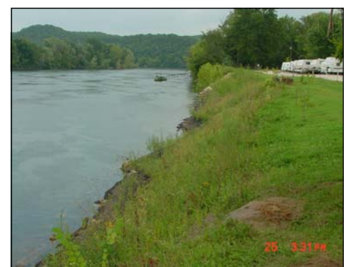
Stabilized bank one year after restoration.
