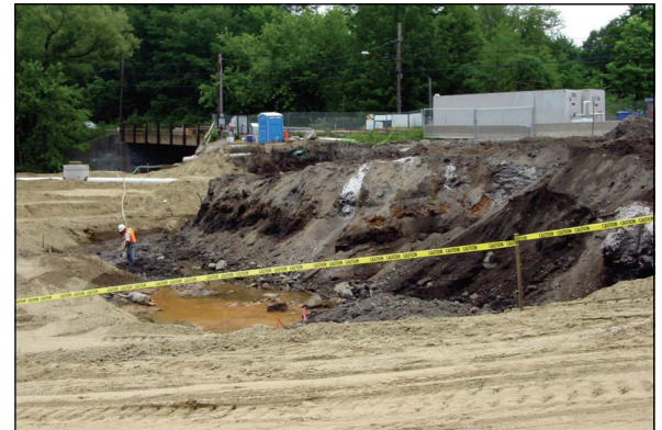
Removal of coal tar deposits from the isolated pond.
