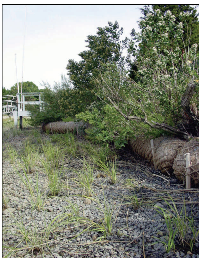
Coir fascines, with adjacent Spartina alternifolia plantings.
