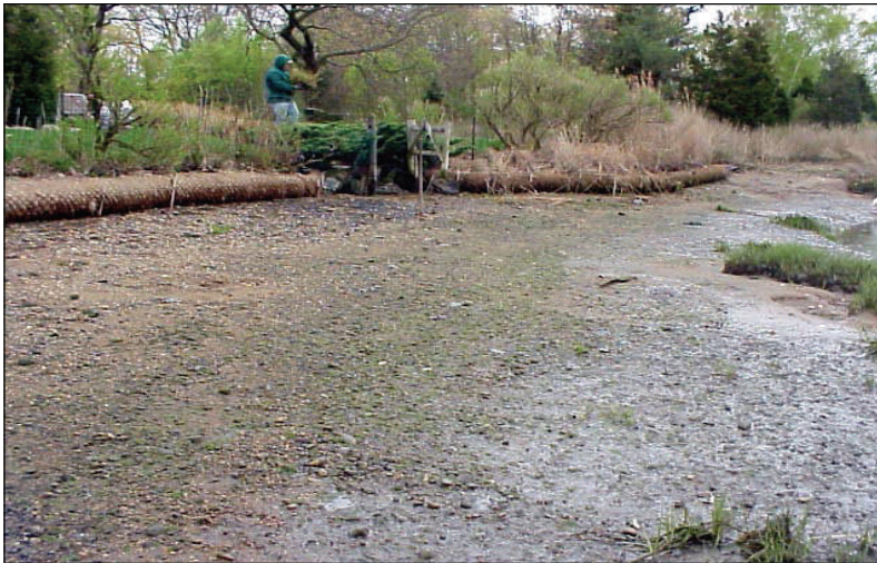
Existing conditions prior to replanting Spartina alternifolia . The coir fascines installed along the bank by NEE are visible in this photograph.
