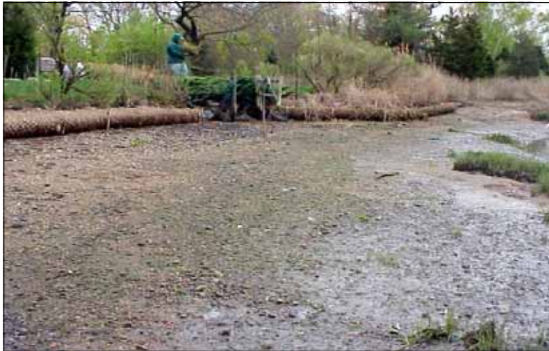
Existing conditions prior to replanting Spartina alternifolia . The coir fascines installed along the bank by NEE are visible in this photograph.
