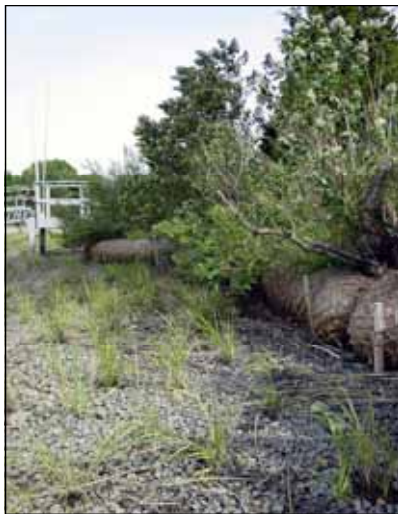
Coir fascines, with adjacent Spartina alternifolia plantings.
